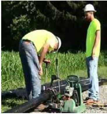
Figure 3: Example of butt fusion
