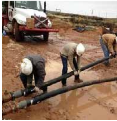
Figure 4: Example of electrofusion
