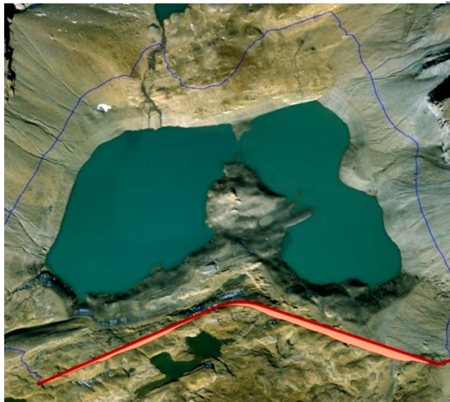
Linthal 2015 – Muttssee Dam (H = 36 m), Upper Reservoir, Switzerland
