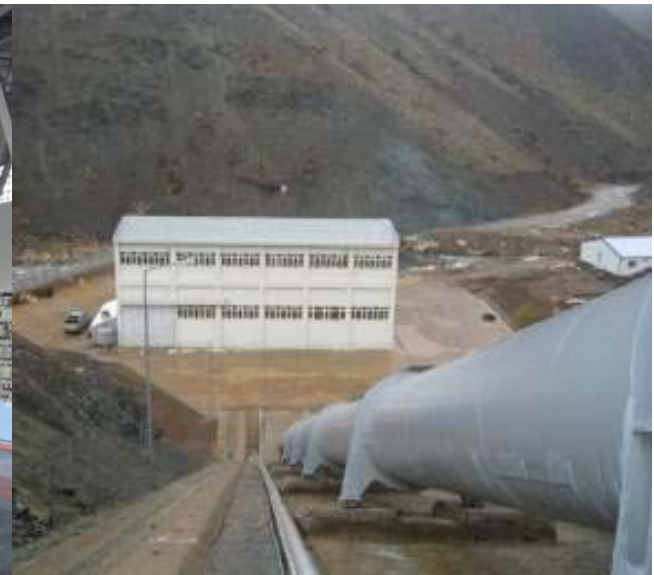
Zorlu / Rehabilitation and upgrading of 7 Hydropower Plants, Turkey
