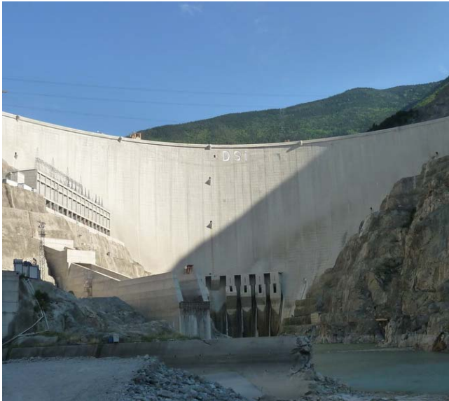
Deriner Dam & HEPP (H = 249 m), Turkey
