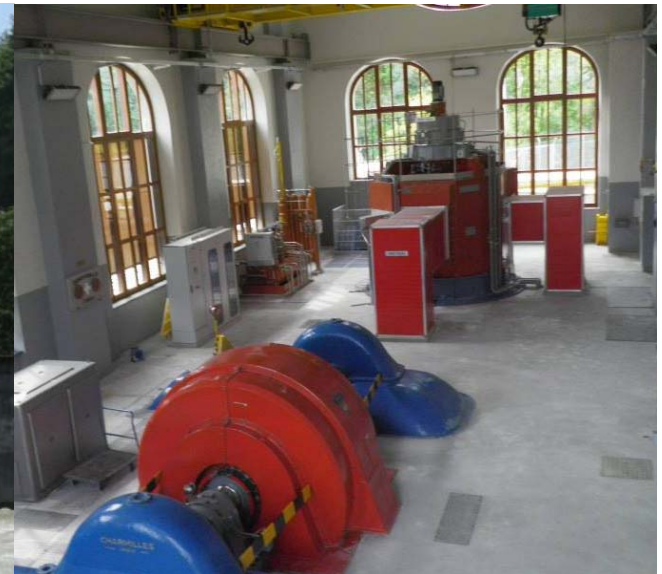
Vièze Hydroelectric Powerhouse Rehabilitation / Unit 1, Switzerland
