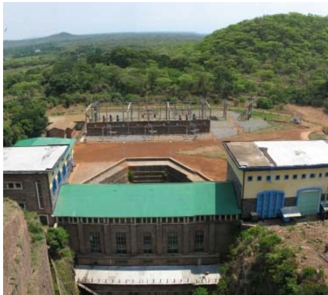
Rehabilitation of Koni Hydropower Plant (42 MW), DR Congo
