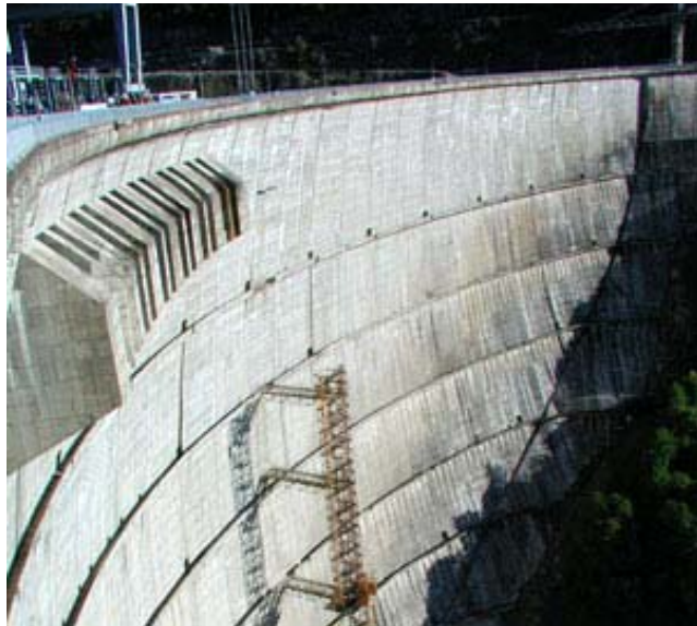
Enguri Dam & HEPP rehabilitation, Georgia
