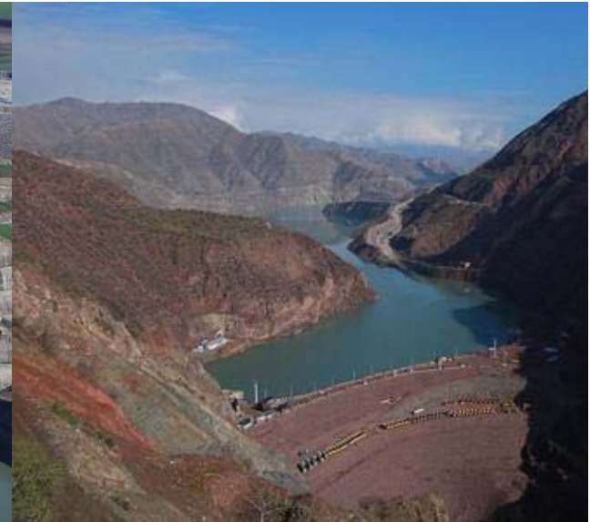
Rogun Dam & hydropower scheme (H = 335 m), Tajikistan
