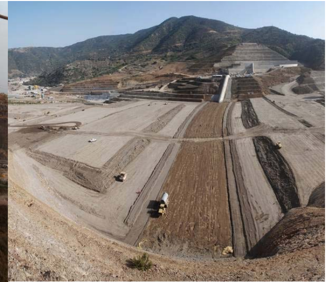
Kef Eddir Earthfill Dam (H = 95 m), Algeria
