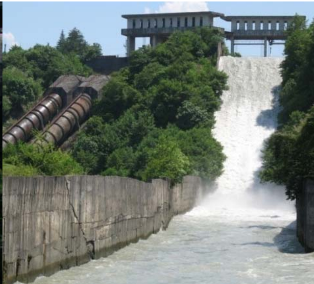
Vardnili Cascade Rehabilitation Project (340 MW), Georgia
