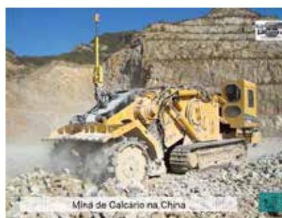
Figure 4 - Surface Miner T1255 - Vermeer Mine of Limestone - China. Source: Vermeer 2014
