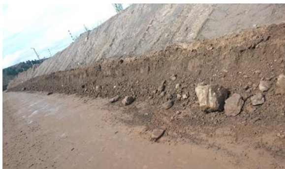
Figure 5 – Blocks moved to the foot of the side windrow access.
