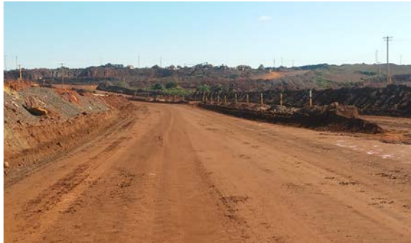
Figure 4 – Part of the road where windrow corners and roads were cleared.
