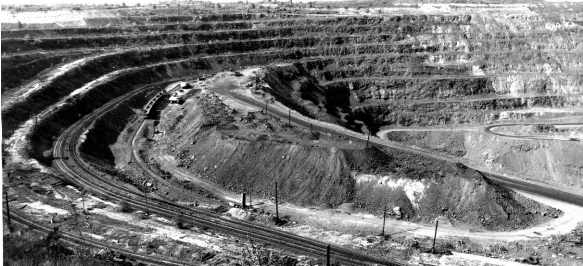
Figure 2 - Excavator operated dumping station on an open pit mine
