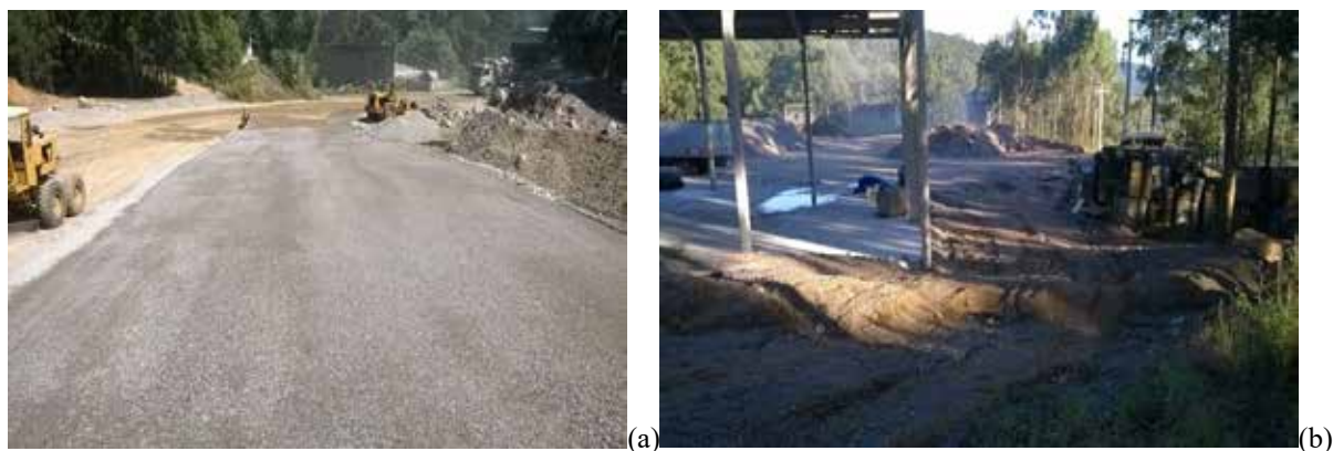
Figure 8: New haul road (a) and previous access (b)
