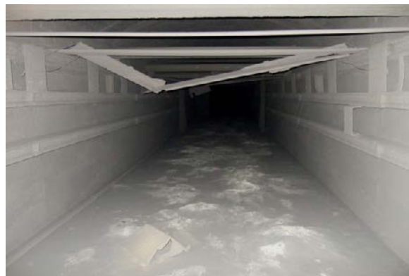
Photo 13. Stone dust barrier with tanks placed in an experimental heading at 400 m. after explosion
