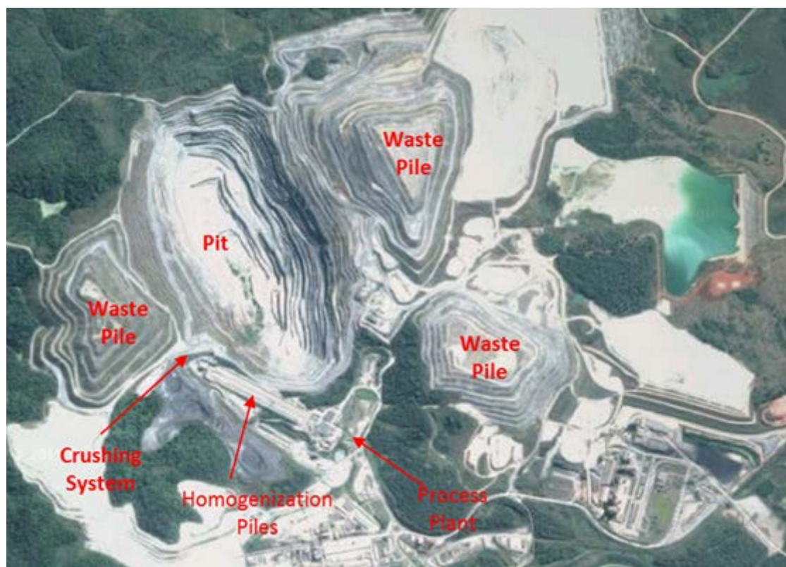
Figure 2 - Overall view of the pit location and the surrounding surface structures
