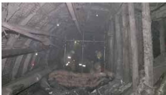
The crew placing sacks
