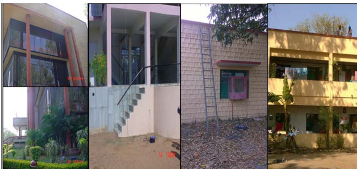
Photograph 1. Monitoring of response of reinforced concrete structure to blast induced vibration.
