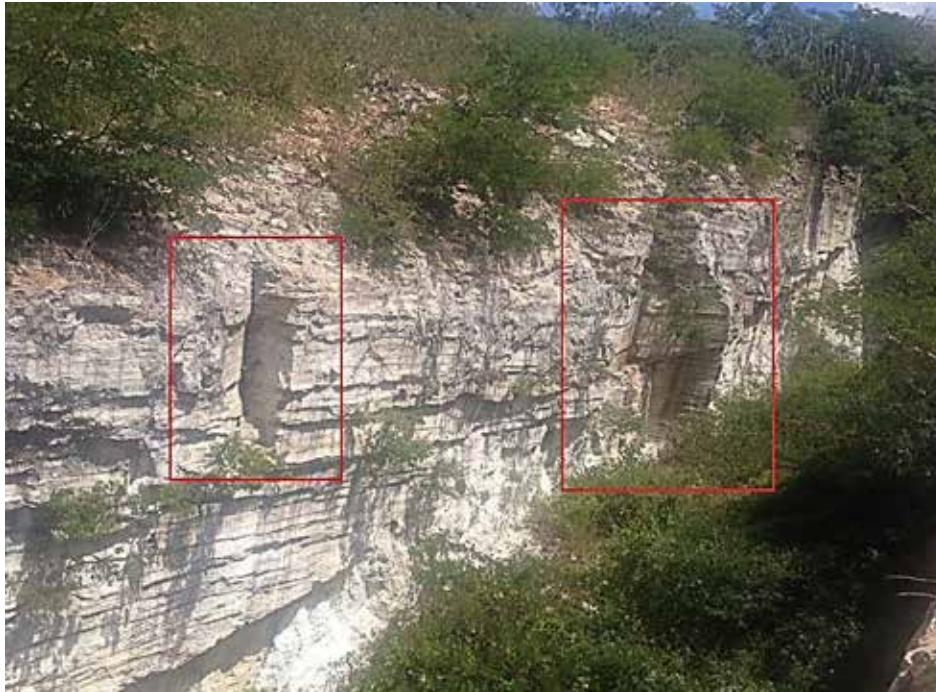
Figure 7 – Wedge failed at opening 1
