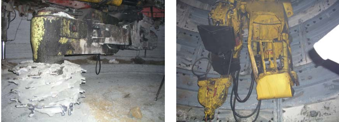
Figure 3 – Mechanical miner (left) and shaft mucker (right)
