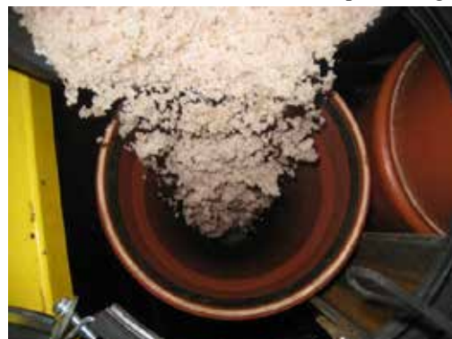
Fig. 8 Installation of the material
