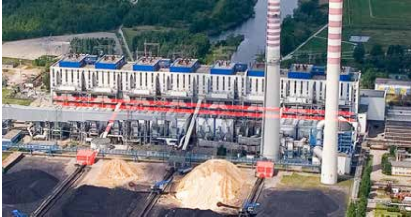
Photo 7. The Dolna Odra Power Plant, the course of explosion
