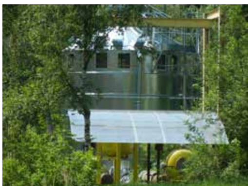
Photo 5. Grain silo of the volume 136 m 3
