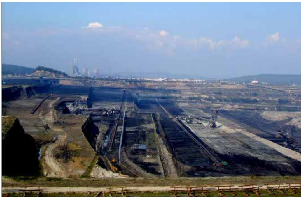
Figure 3. Continuous flow technology – Rosia coal pit from Oltenia [5].
